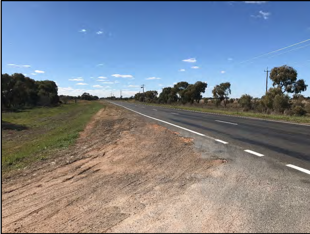
Photo 2 – View to left for drivers exiting Ercildoune Road onto the Kidman Way
