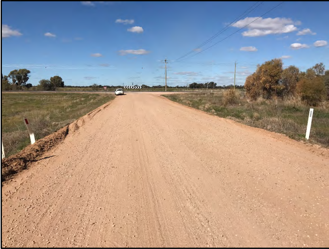
Photo 4 – Typical cross section for the Ercildoune Road
