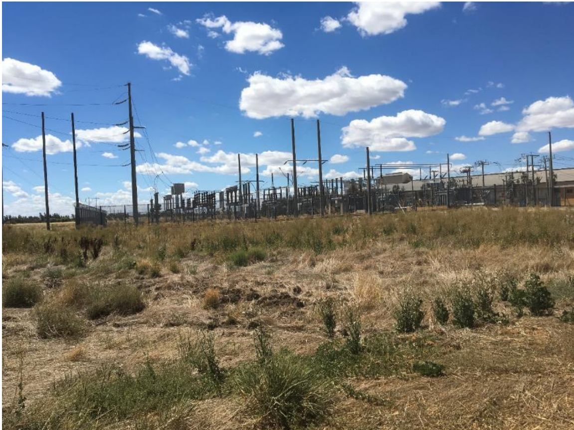
Figure 3-5 Existing substation accessed from Ercildoune Road.
