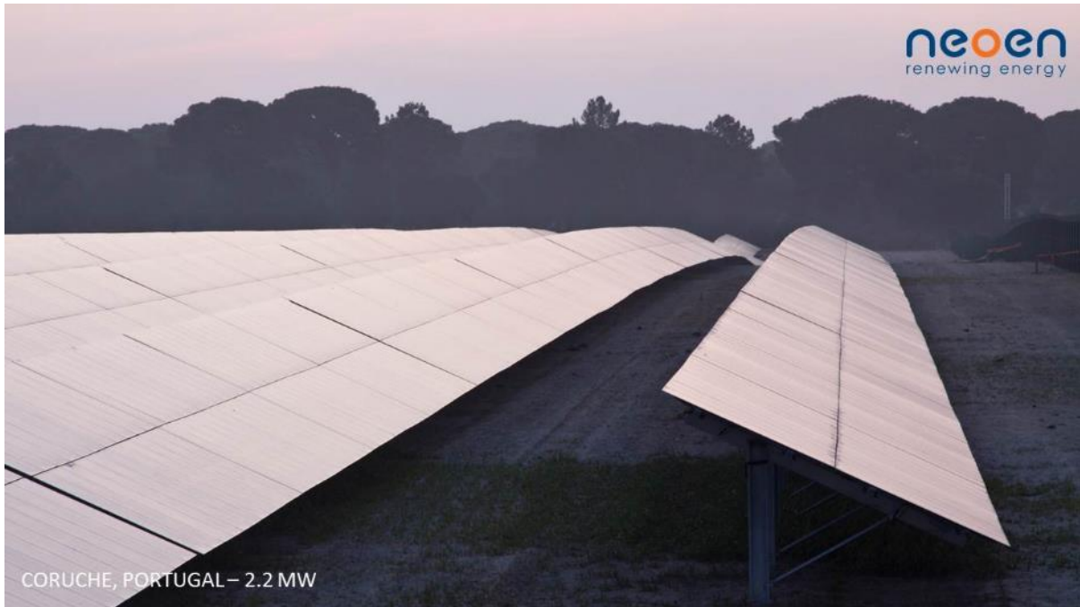
Figure 2-2 Example of south-facing fixed-tilt mounting system with thin-film technology in Europe (installation in Australia would face the north)
