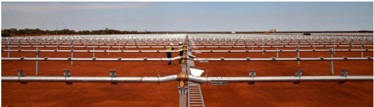
Figure 3-7 Example of a single-axis mounting system before panel installation
